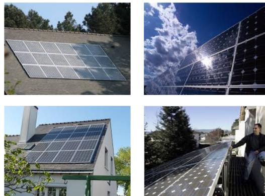
Fig 3: Shading on photovoltaic arrays.
